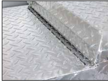
Fully concealed aluminum continuous hinge.
